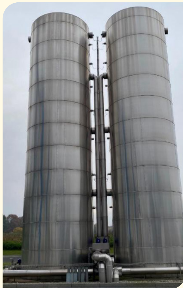
— Schne-frost heat recovery system to produce hot water
